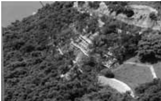
Installation of soil nails, erosion control mat and wire mesh, maintenance stairway
